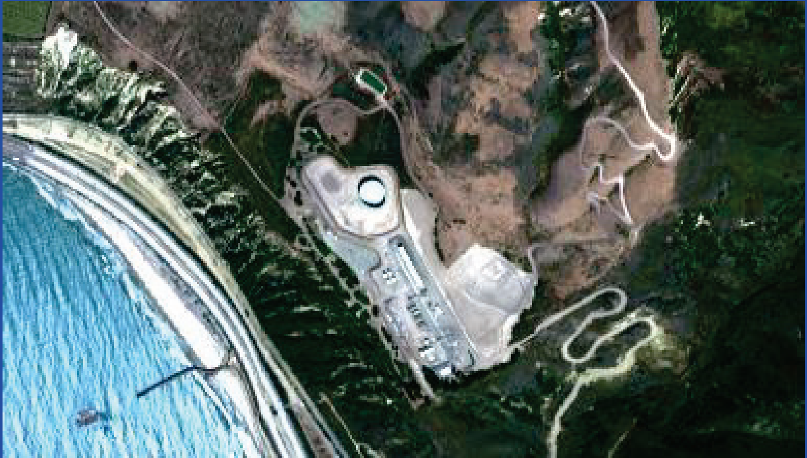
Pumping Facility in terrain characterized by oil seeps....
